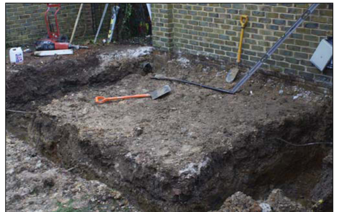
Plate 4. General view of excavated footing trenches, looking South east.
