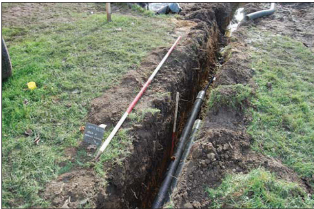
Plate 7. Area A, service trench, looking south east, Scales: 2m and 1m.
