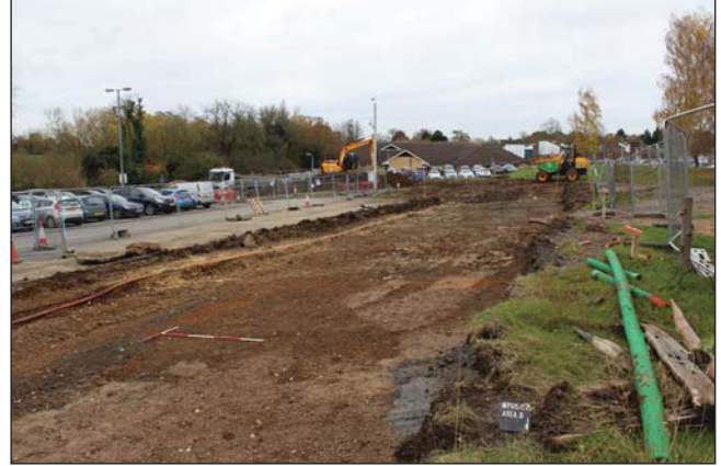
Plate 10. Area D, looking southeast, Scales: 2m and 1m.
