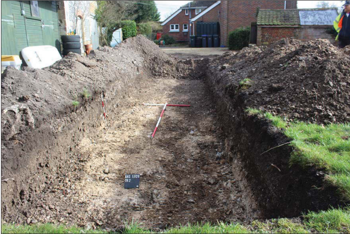
Plate 5. Trench 2, Removal of made ground(55), looking east. Scales: 2m, 1m and 0.5m
