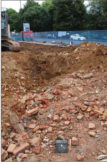
Plate 1. Site excavations, looking north east.
