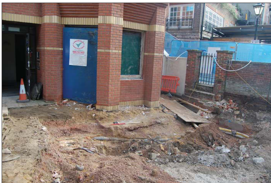
Plate 2. Site, looking south, Scale: 1m.
