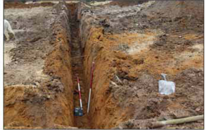
Plate 2. Southern footing trench, looking East. Scales: 2m and 1m.
