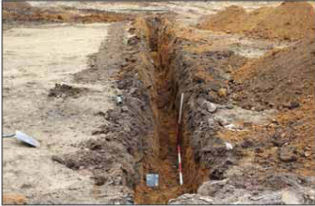
Plate 1. Western footing trench, looking South. Scales: 2m and 1m.
