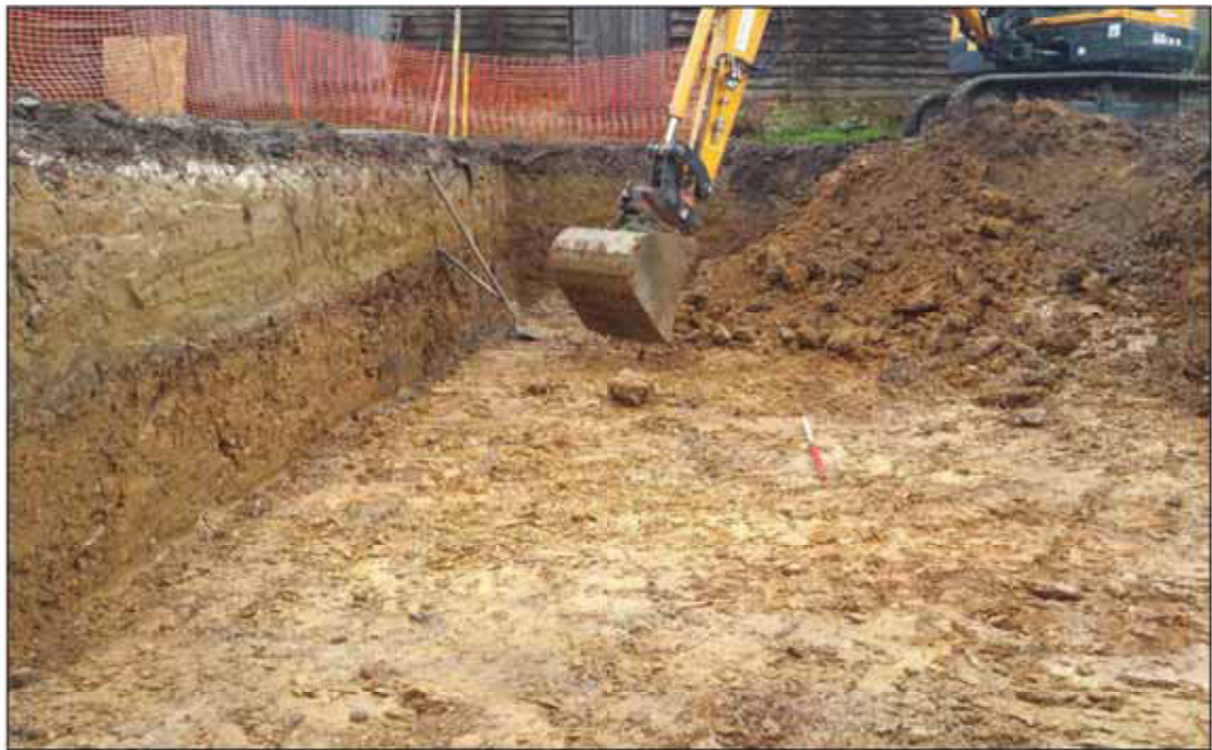
Plate 4. Base of excavation, looking east north east, Scale: 1m.
