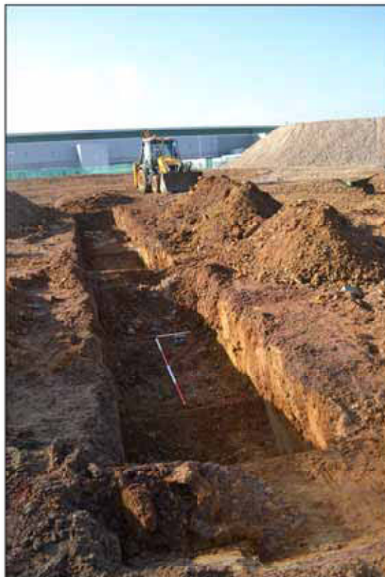
Plate 5. Trench 8, looking NE, Scales: 2m, 1m and 0.5m.
