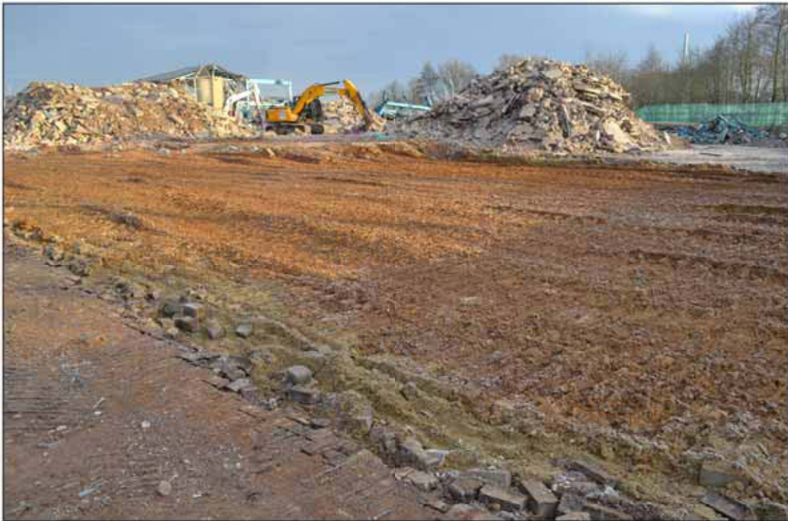
Plate 1. After demolition, prior to trenching, looking north east.
