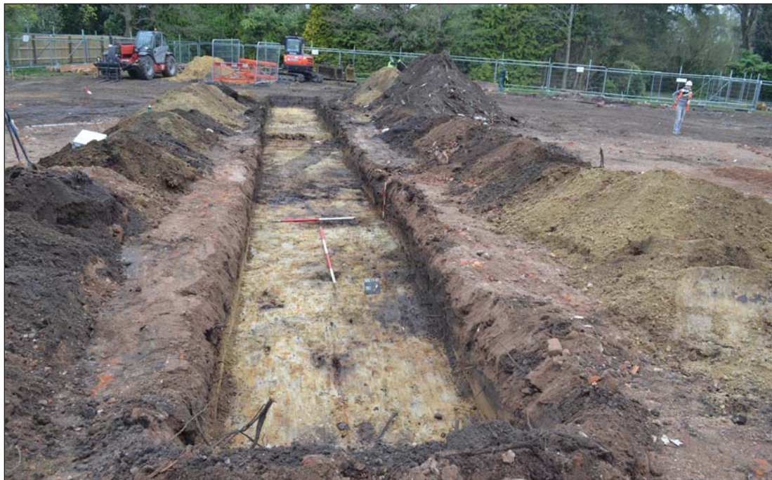
Plate 2. Trench 2, looking north west, Scales: horizontal 2m and 1m, vertical 0.5m.
