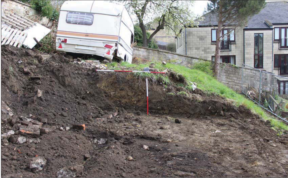
Plate 1. Deposits 50, 51 and 52 under excavation. Looking East Scales: 2m and 1m
