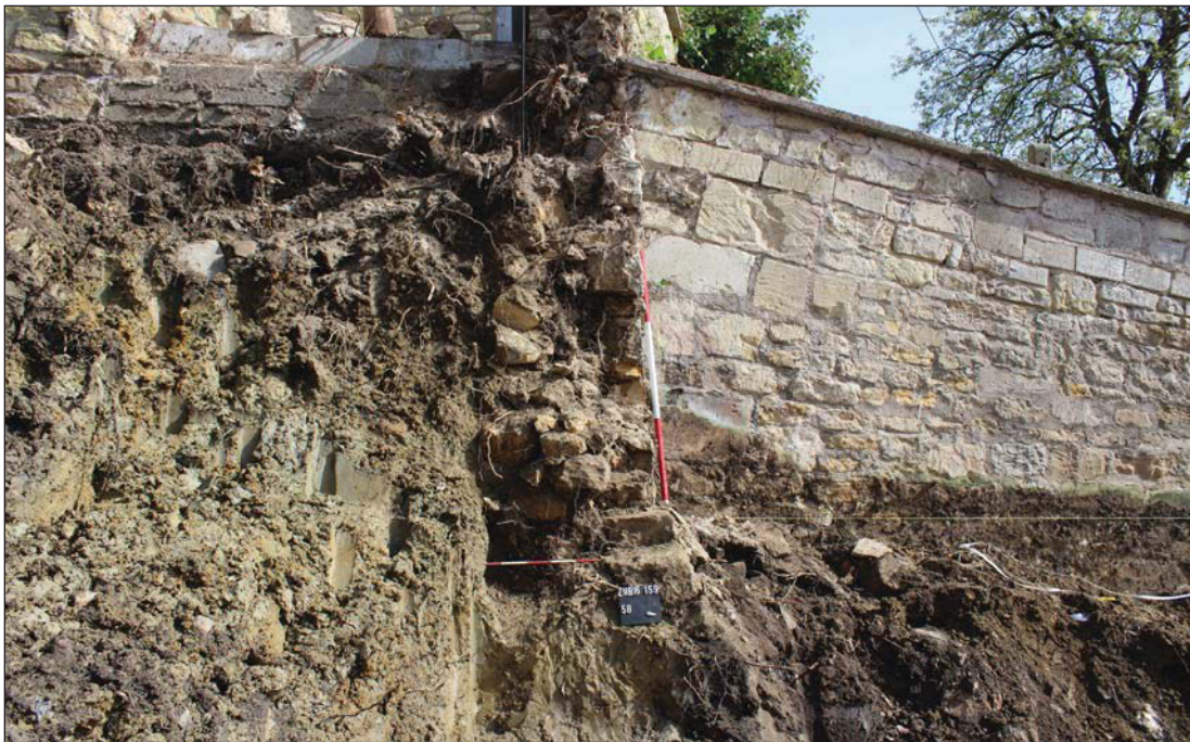
Plate 2. Wall 58 Cut 2 looking East. Scales: 2m and 0.5m
