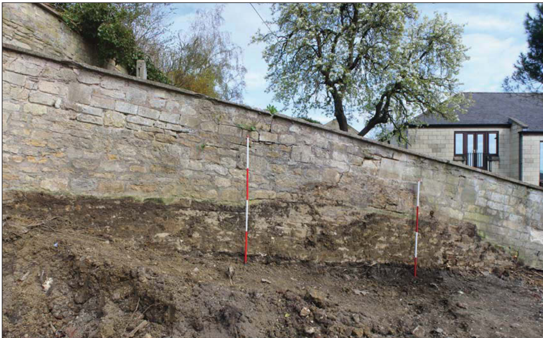
Plate 4. Wall 57 Looking East Scales: 2m and 2m
