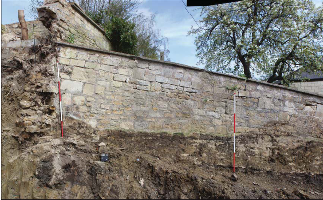
Plate 3. Walls 57 and 58 Cuts 2 and 3 Looking East, Scales: 2m and 2m
