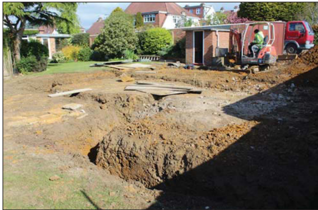
Plate 3. General view of site, looking North-west.
