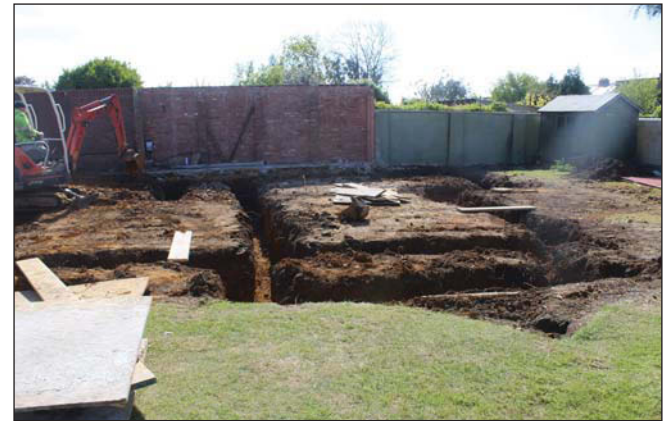
Plate 4. General view of site, looking East.
