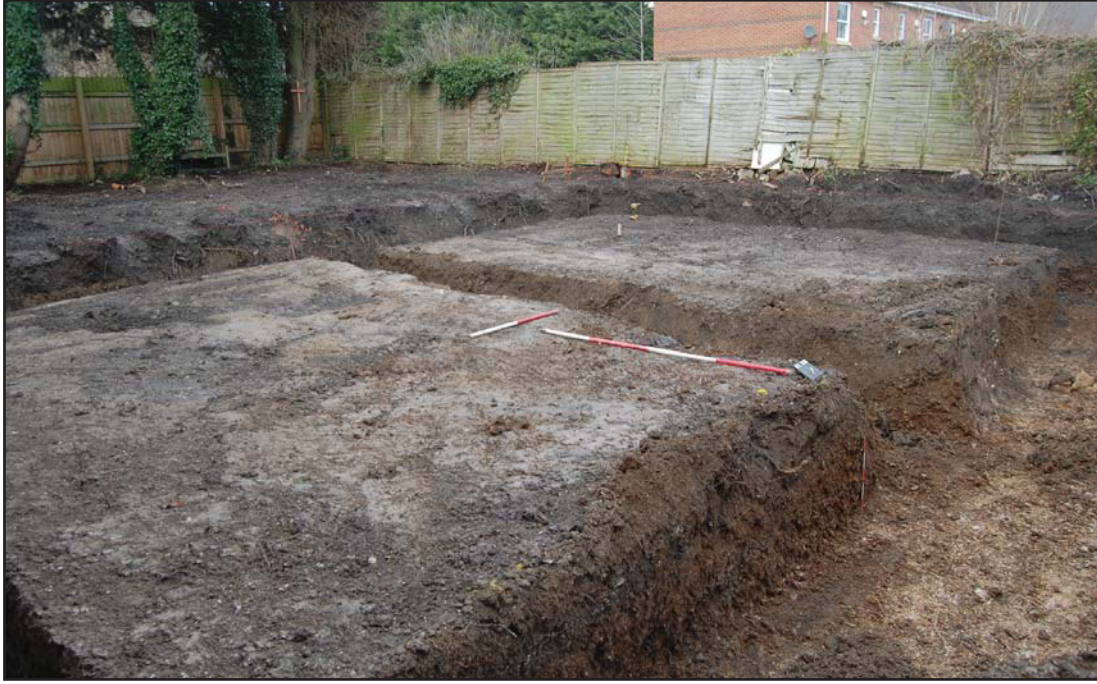
Plate 1. Footing trenches, looking North, Scales: 2m, 1m and 0.5m.
