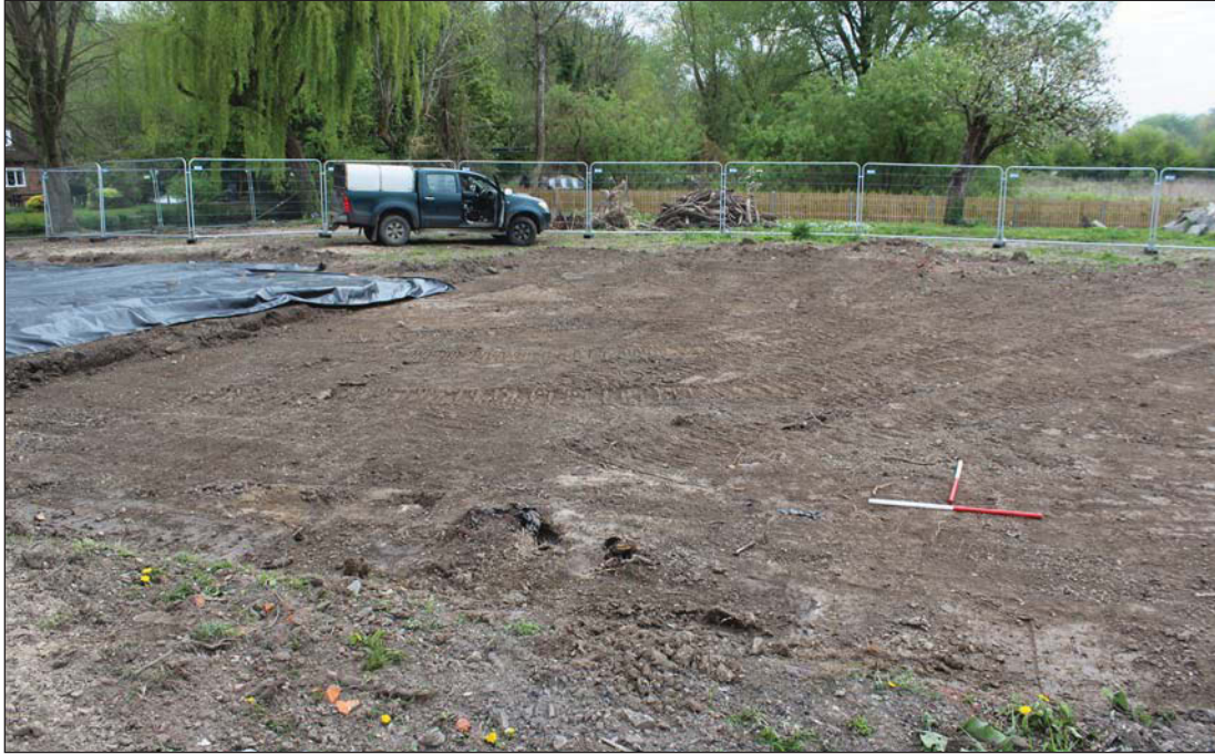
Plate 1. View over stripped area on east of site, looking east, Scales: 2m and 1m.
