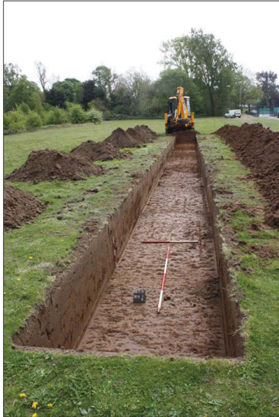
Plate 3. Trench 10, looking south, Scales: horizontal 2m and 1m, vertical 0.5m.
