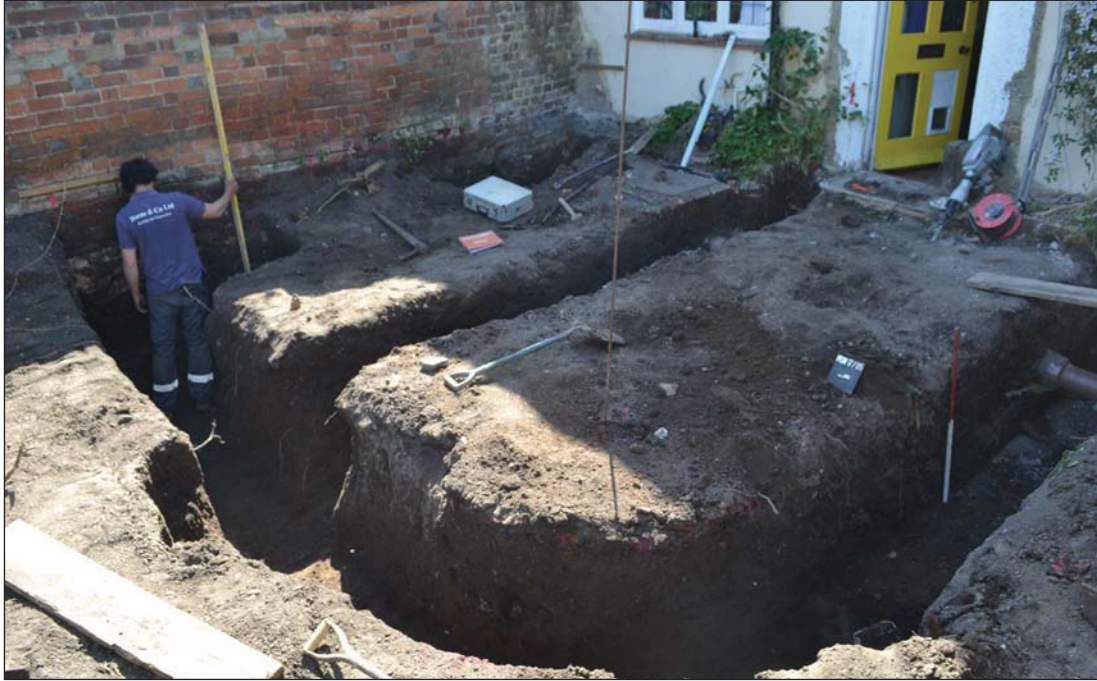
Plate 1. Extension footings after excavation, looking south west, Scale: 1m.
