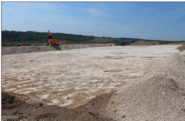
Plate 3. General view of Northern Area, looking South-west.
