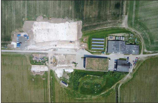
Plate 1. Aerial view of site taken during groundworks.
