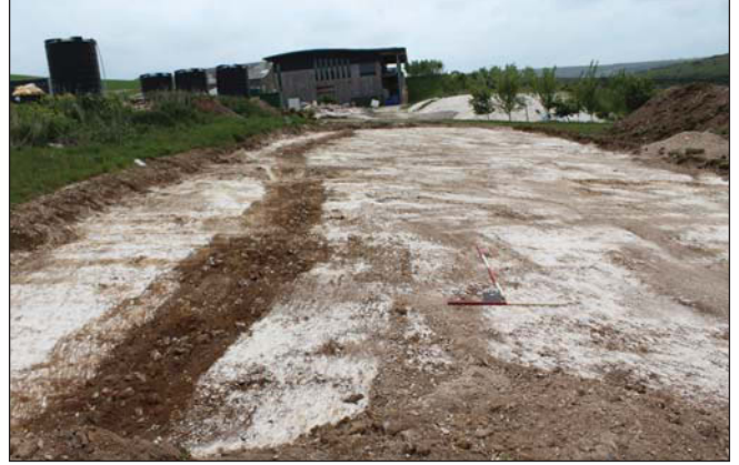
Plate 6. General view of Southern Area, looking East. Scales: 2m and 1m.
