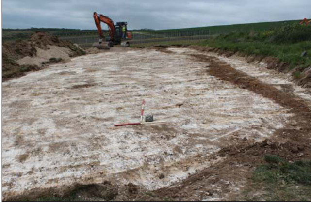
Plate 5. General view of Southern Area, looking West. Scales: 2m and 1m.
