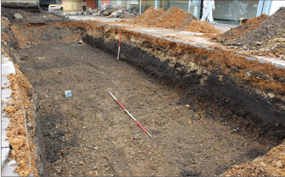
Plate 1. Trench 1, looking north west. Scales: 2m and 1m.
