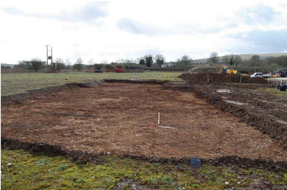
Plate 1. Area of strip, looking south west, Scales: 2m and 1m.
