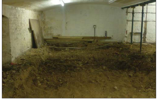
Plate 2. General view of south-west corner of interior, looking North-west.
