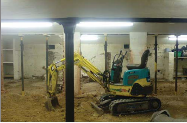
Plate 1. General view of interior, looking North-east.
