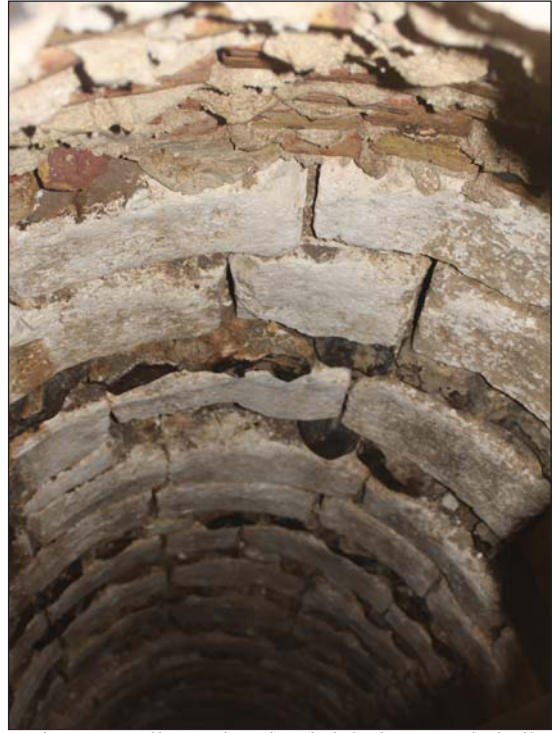
Plate 6. Well 51, showing brick dome and chalk block lining.
