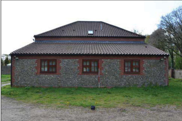
Plate 5. Exterior, side extension, looking southeast, Scales: 2m.
