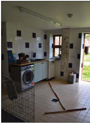
Plate 9. Interior, room 2, utility room, looking north, Scales: 2m and 1m.
