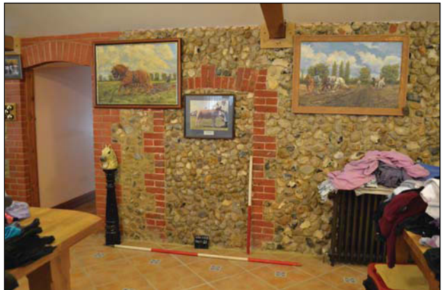
Plate 12. Interior, room 4, blocked door, looking southeast, Scales: 2m and 1m.
