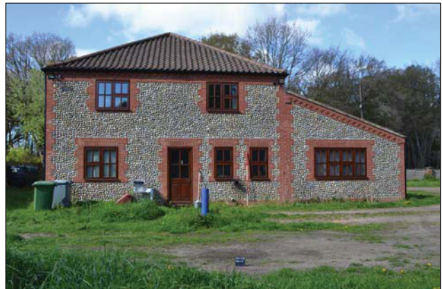
Plate 4. Exterior, rear elevation, looking southwest, Scales: 2m.
