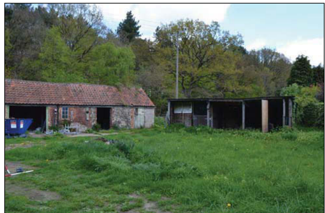
Plate 20. Exterior, outbuildings, looking northeast, Scales: 2m and 1m.
