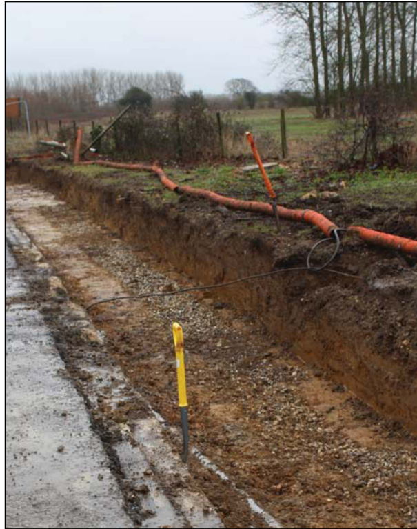
Plate 5. General view of Mitigation Area B, looking East.
