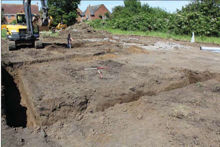
Plate 2. Excavation of garage footing, looking north east, Scales: 1m x2.
