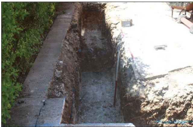
Plate 3. Southern footing trench, looking West. Scales: 2m and 1m.
