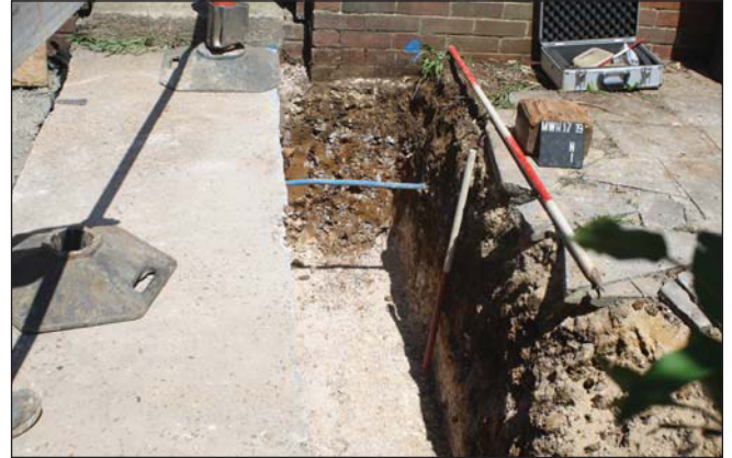
Plate 2. Western footing trench, looking North. Scales: 2m and 1m.
