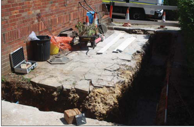
Plate 5. General view, looking East.
