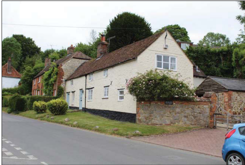
Plate 1. The Grade II Listed property 12 Oxford Street, looking south east.
