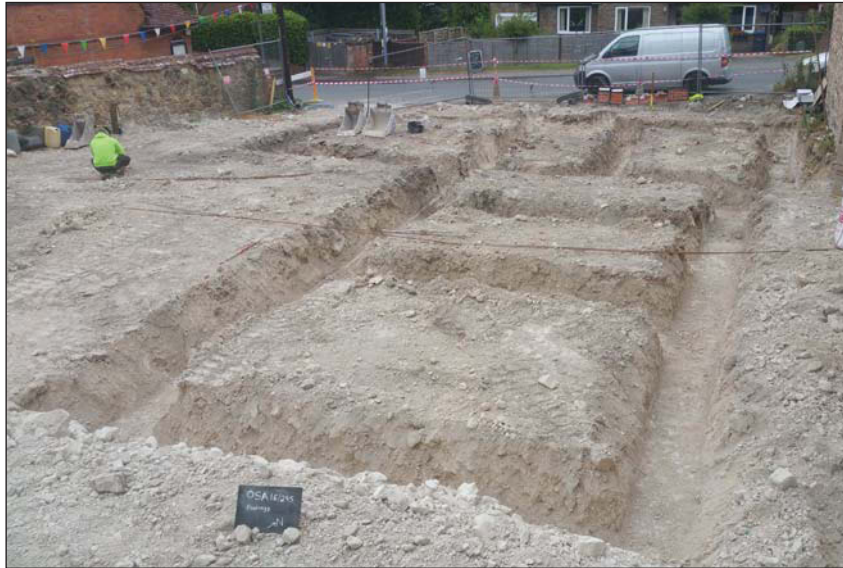
Plate 3. The excavated footings, looking north west.
