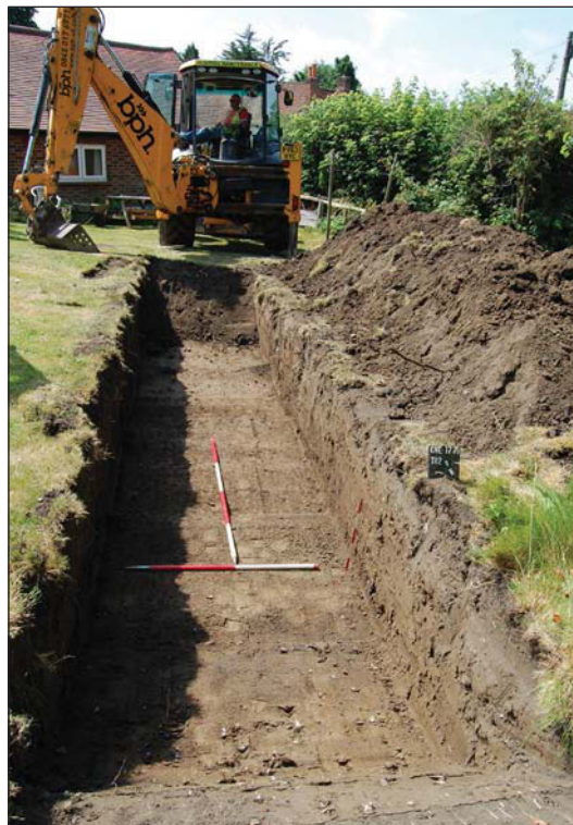
Plate 2. Trench 2, looking south west, Scales: horizontal 2m and 1m, vertical 0.5m.
