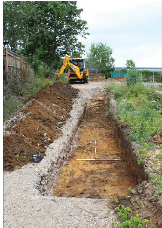
Plate 4. Trench 4, looking east, Scales: horizontal 2m and 1m, vertical 0.3m.
