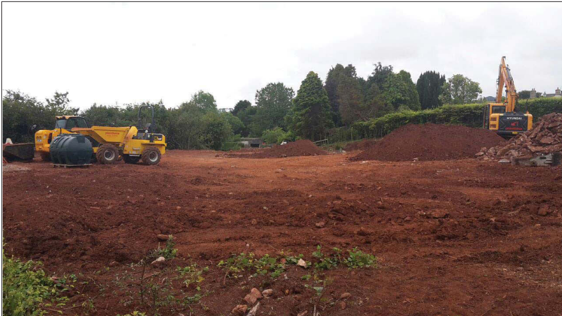
Plate 4. General view of site during overburden stripping.
