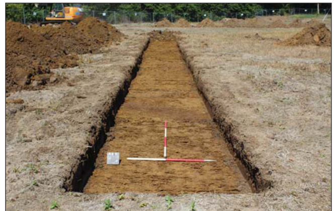
Plate 8. Trench 32, looking North-west. Scales: 2m, 1m and 0.30m.
