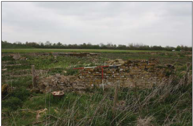
Plate 4. External face of west wall, looking north east, Scales: 2m and 1m.
