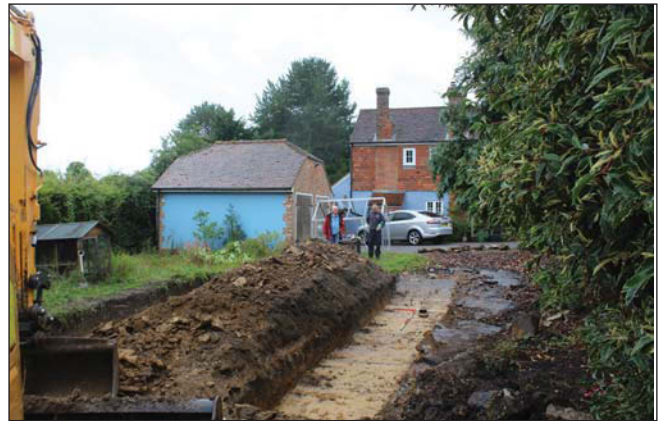
Plate 4. General view, looking South.
