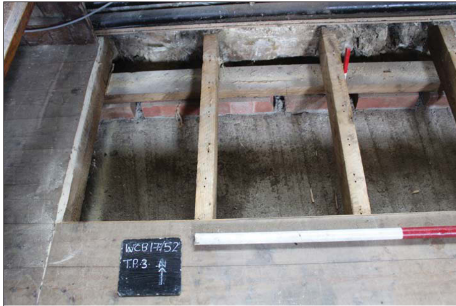
Plate 3. Interior, test pit 3, looking north, Scales: 1m and 0.3m.
