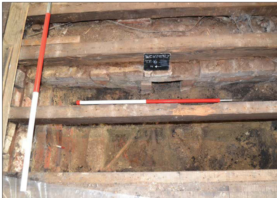
Plate 4. Interior, test pit 4, looking north, Scales: 1m x2.
