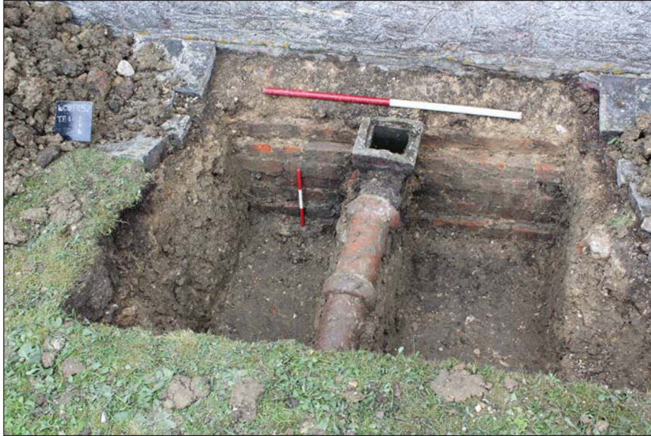
Plate 1. Exterior, test pit 1, looking south, Scales: 1m and 0.3m.
