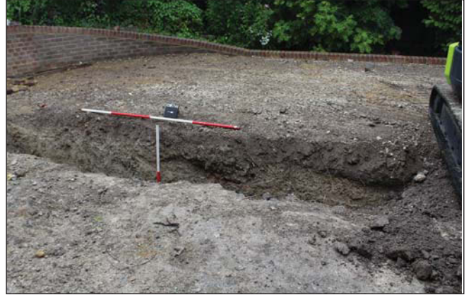
Plate 2. Western footing trench, looking West. Scales: 2m and 1m.
