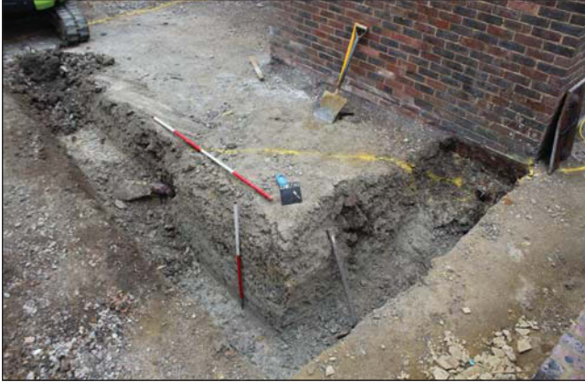
Plate 1. Southern end of footings, looking North-east. Scales: 2m and 1m.
