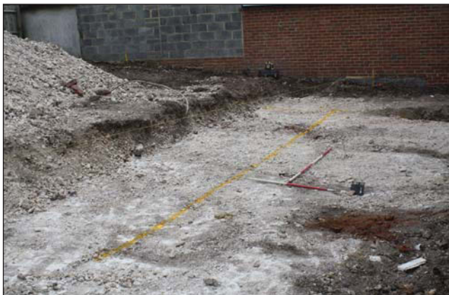
Plate 3. General view of stripped area, looking South. Scales: 2m and 1m.
