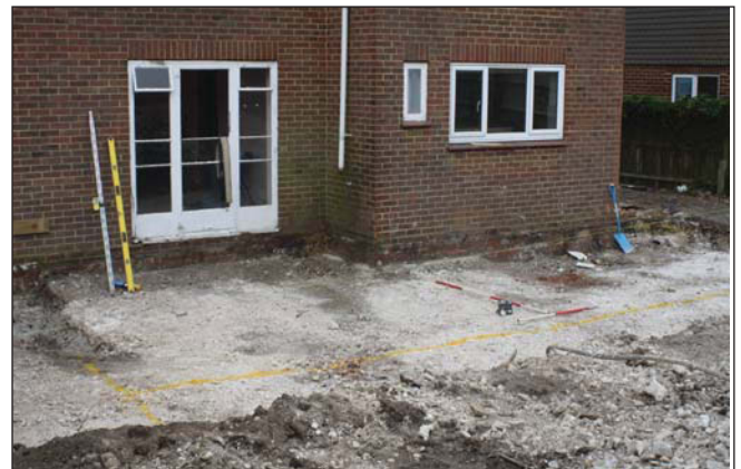
Plate 4. General view of stripped area, looking West. Scales: 2m and 1m.
