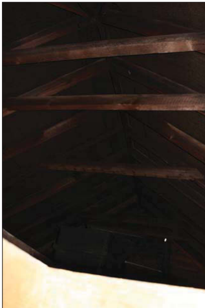
Plate 30. Room 1, roof detail, looking southeast.
