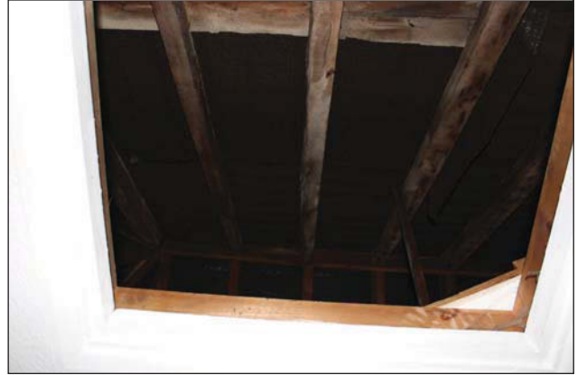
Plate 21. Room 10, roof space, looking east.
