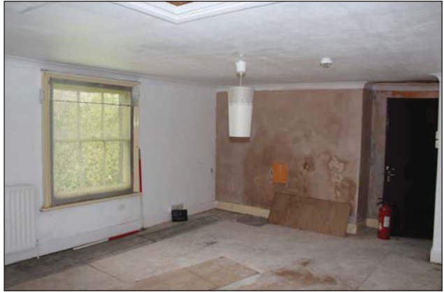
Plate 29. Room 1, looking northwest, Scales: 2 x 1m.
