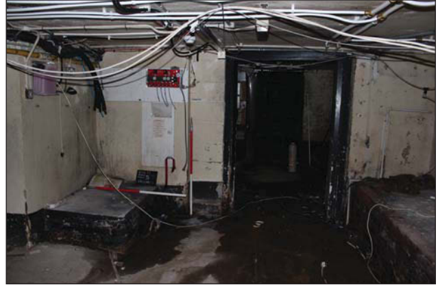
Plate 13. Room 27, looking northeast, Scales: 2 x 1m.
