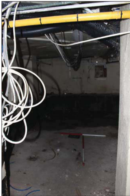
Plate 14. Room 28, looking northwest, Scales: 2 x 1m.
