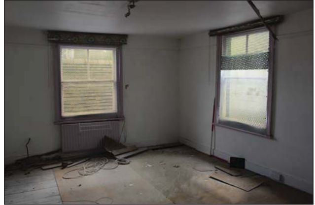
Plate 19. Room 2 looking east, Scales: 2 x 1m.
