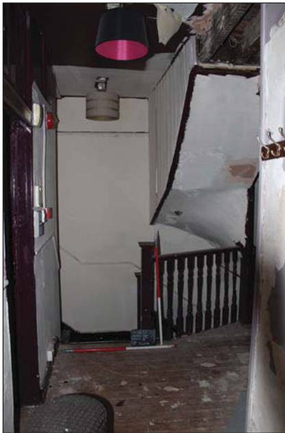
Plate 6. Corridor 4, towards stairs, looking east, Scales: 2 x 1m.
