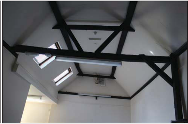
Plate 33. Room 16, truss, looking southwest.
