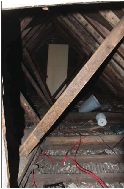
Plate 12. Phase 1 roof detail, looking northwest.
