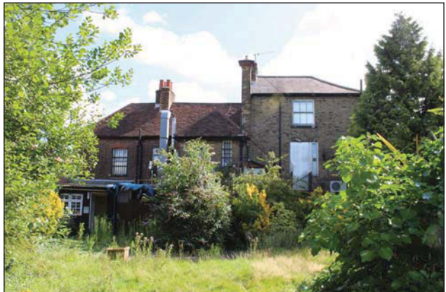
Plate 3. Rear of the building, looking northeast.
