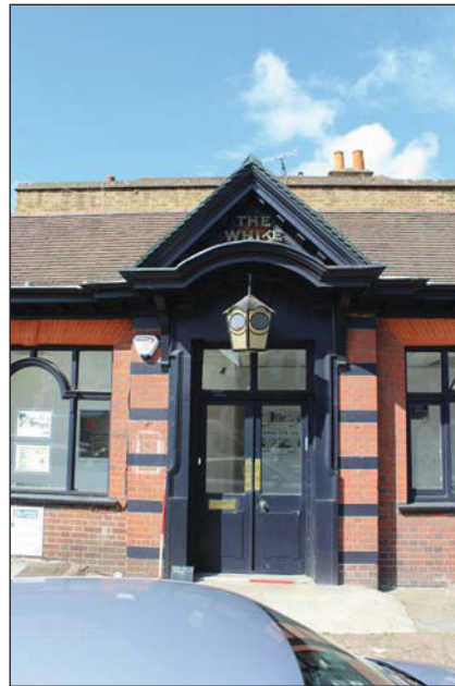
Plate 35. Main entrance, looking southwest, Scales: 2 x 1m.
