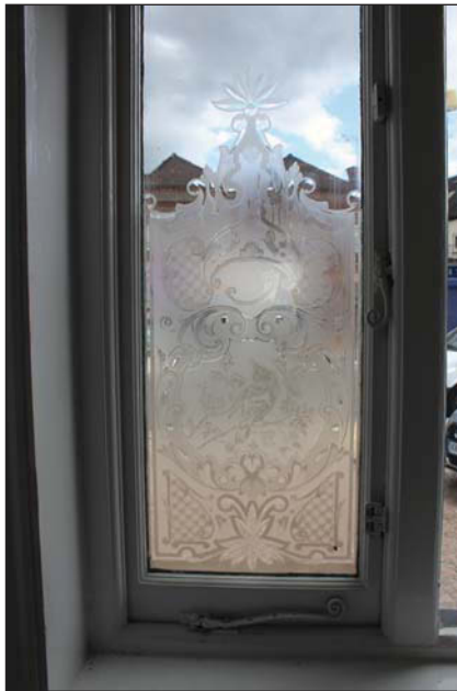
Plate 34. Room 22, window detail, looking northeast.
