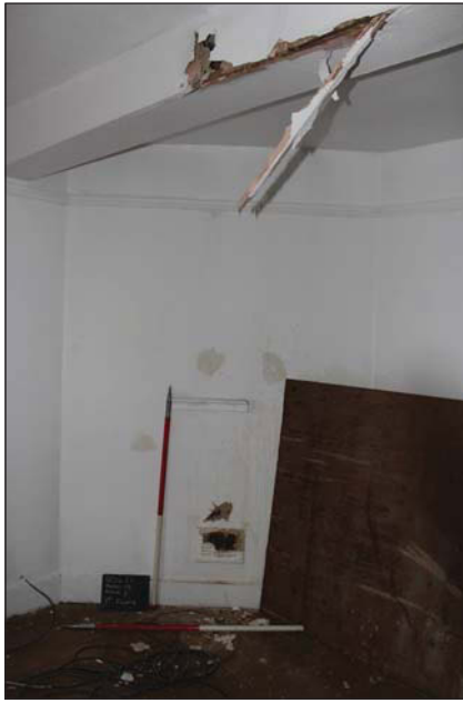
Plate 20. Room 2, to chimney breast, looking southwest, Scales: 2 x 1m.
