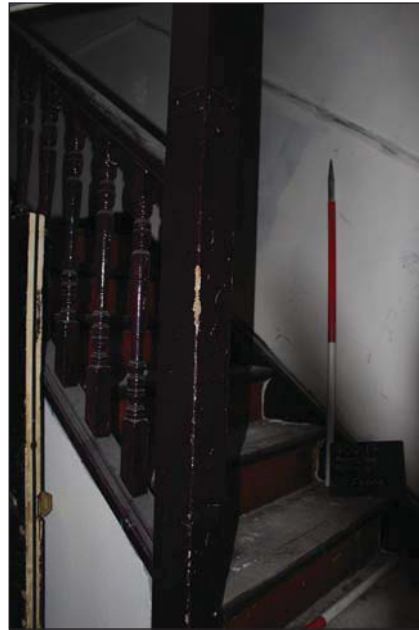
Plate 25. Room 8, stair detail, looking northwest, Scales: 2 x 1m.
