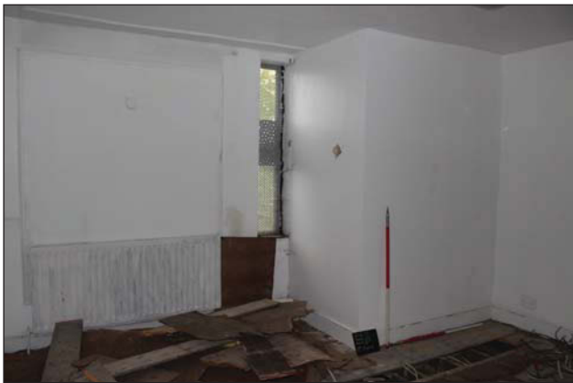
Plate 26. Room 3, looking northwest, Scales: 2 x 1m.
