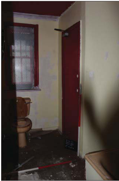
Plate 28. Room 5, looking west, Scales: 2 x 1m.
