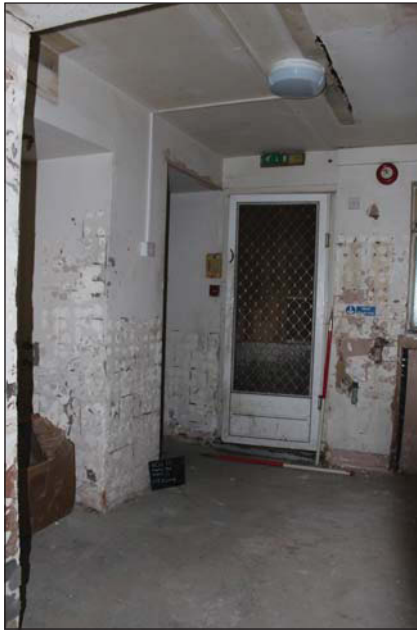
Plate 24. Room 11, looking southwest, Scales: 2 x 1m.
