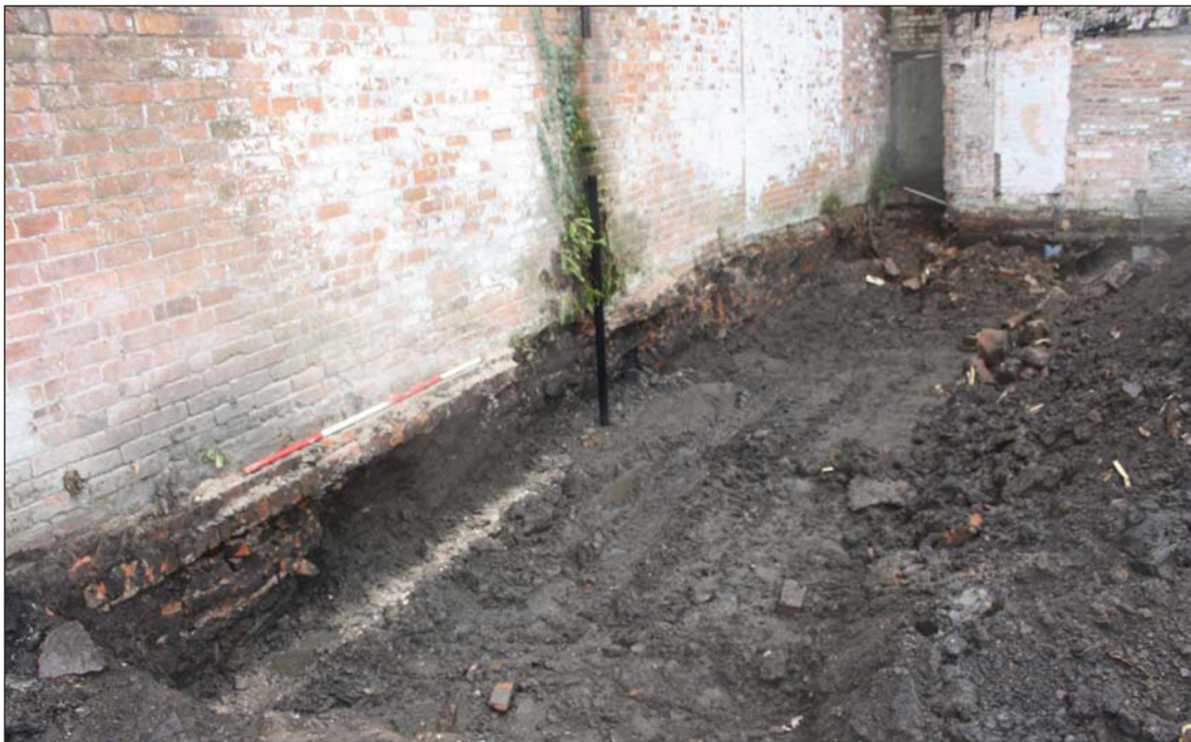
Plate 2. Working shot, looking north, Scale: 2m.
