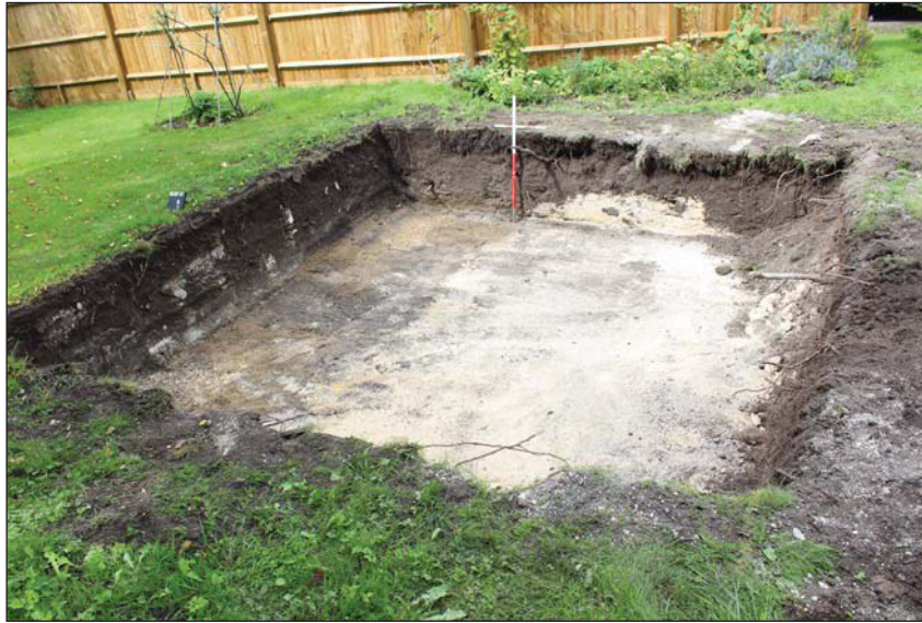
Plate 3. Excavated soakaway trench, looking north, Scales: horizontal 0.5m, vertical 1m.
