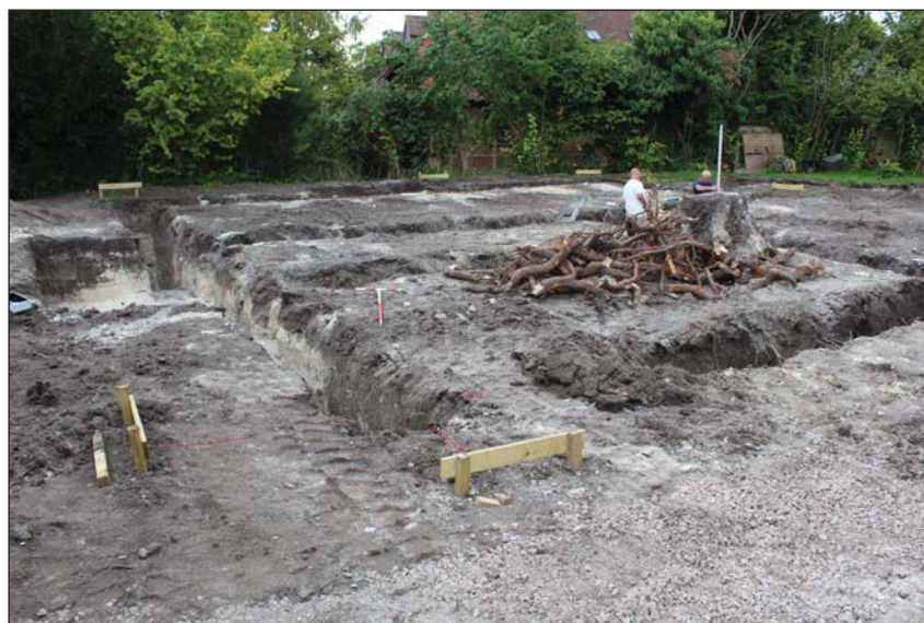
Plate 2. Excavated house footings, looking south, Scales: 1m and 0.5m.
