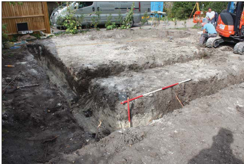
Plate 4. Excavated garage footings, looking east, Scales: 2m and 1m.
