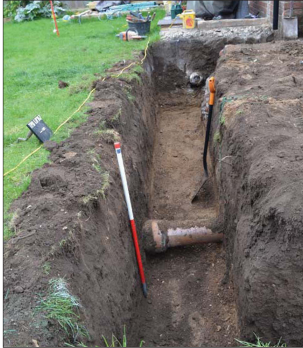
Plate 1. Western footing, looking north, Scale: 1m.
