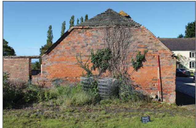
Plate 36. Exterior, east barn gable, looking north, Scales: 2m and 1m.
