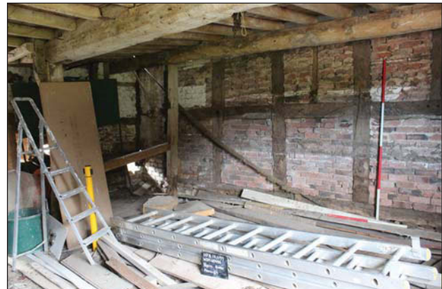
Plate 8. Interior, north barn, Bay 5, looking south west, Scales: 2m and 1m.
