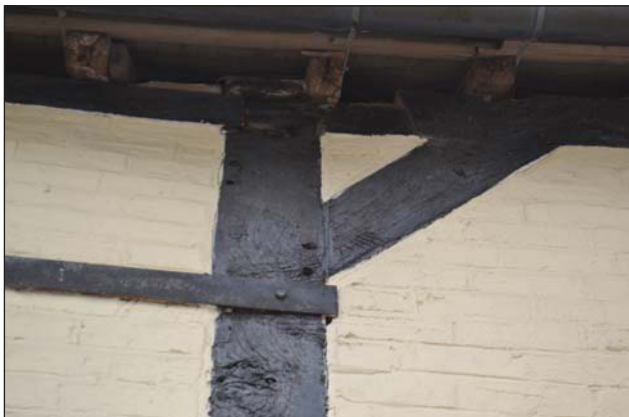
Plate 7. Exterior, detail of beams on north elevation of north barn.
