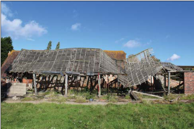
Plate 47. Exterior, south barn, looking north, Scales: 2m and 1m.
