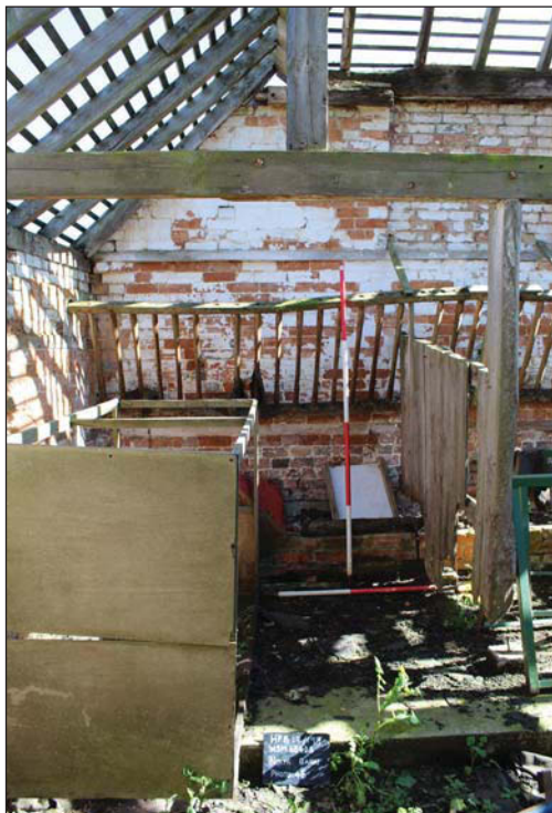
Plate 39. Interior, north barn extension, south wall, Scales: 2m and 1m.
