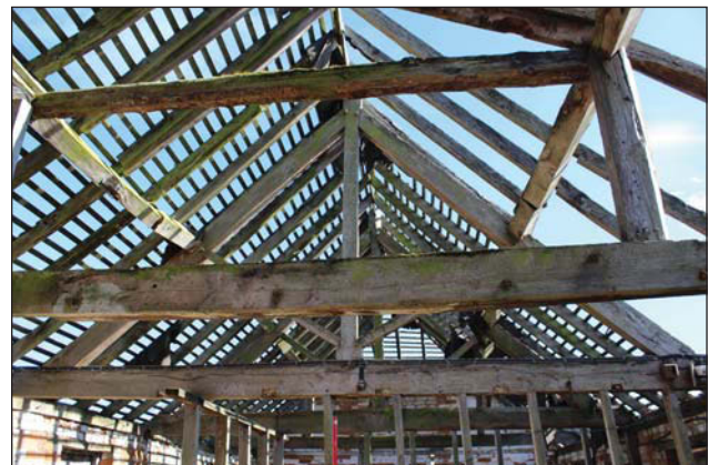
Plate 40. Interior, north barn extension, roof structure, looking north.
