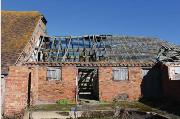
Plate 37. Exterior, Courtyard, north barn extension, west elevation, Scales: 2m and 1m.
