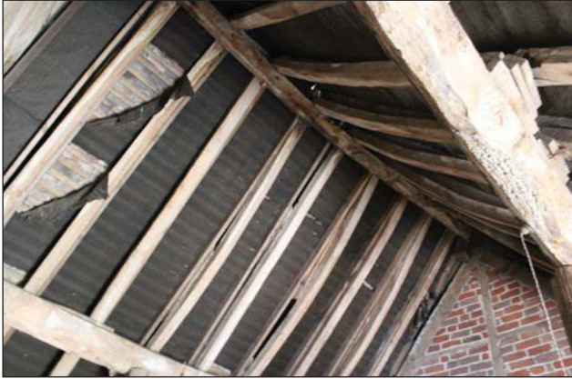
Plate 25. Interior, roof beams from FF2 over Bay 2.
