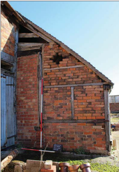
Plate 31. Exterior, Bay 5 lean-to addition, looking east, Scales: 2m and 1m.
