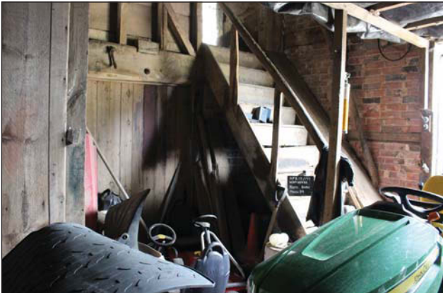
Plate 19. Interior, north barn, Bay 3, looking north west.
