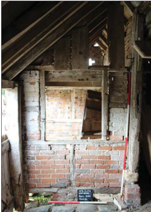
Plate 33. Interior, north barn, east lean-to, looking west, Scales: 2m and 1m.
