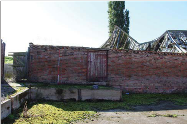
Plate 43. Exterior, south barn, looking south, Scales: 2m and 1m.
