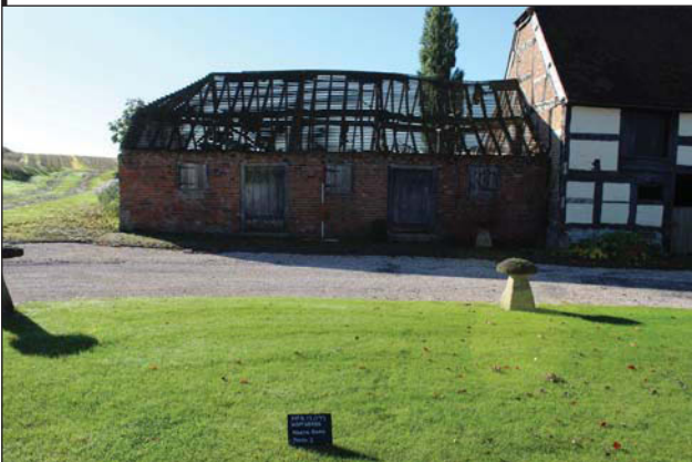
Plate 35. Exterior, east barn, looking west, Scales: 2m and 1m.
