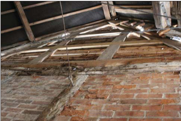
Plate 15. Interior, north barn, western gable from stairs to first floor (FF1).
