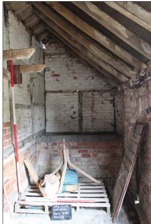
Plate 32. Exterior, north barn, east lean-to, looking west, Scales: 2m and 1m.
