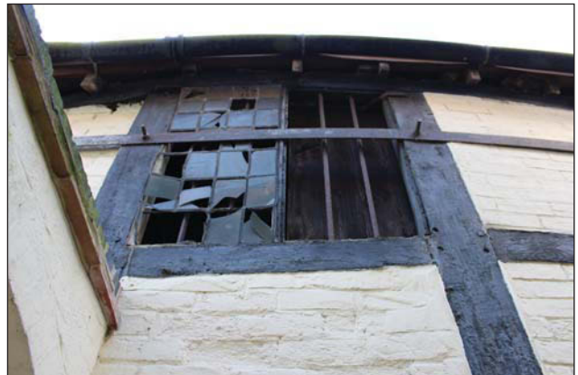
Plate 4. Exterior, north barn, first storey original window condition,
