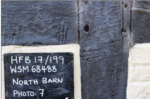
Plate 5. Exterior, carpenters marks of exterior beams.
