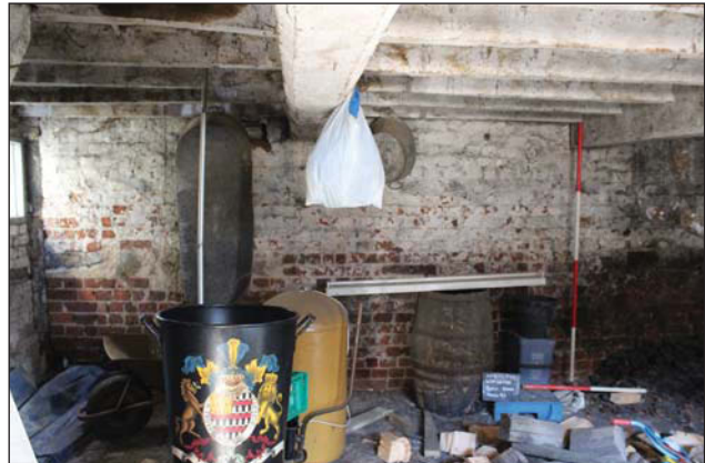
Plate 16. Interior, north barn, Bay 1, looking east, Scales: 2m and 1m.
