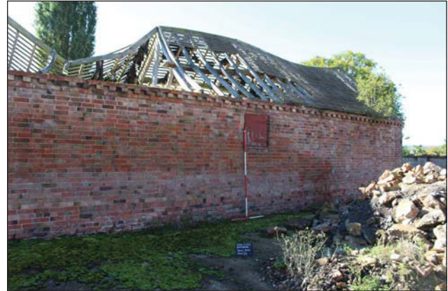
Plate 44. Exterior, south barn, looking south west, Scales: 2m and 1m.
