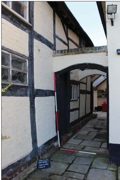
Plate 3. Exterior, entranceway link between Home Farm house and north barn looking west, Scales: 2m and 1m.
