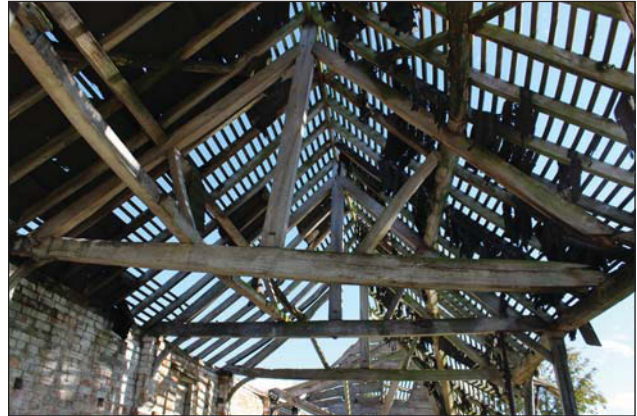
Plate 48. Interior, south barn, roof structure.
