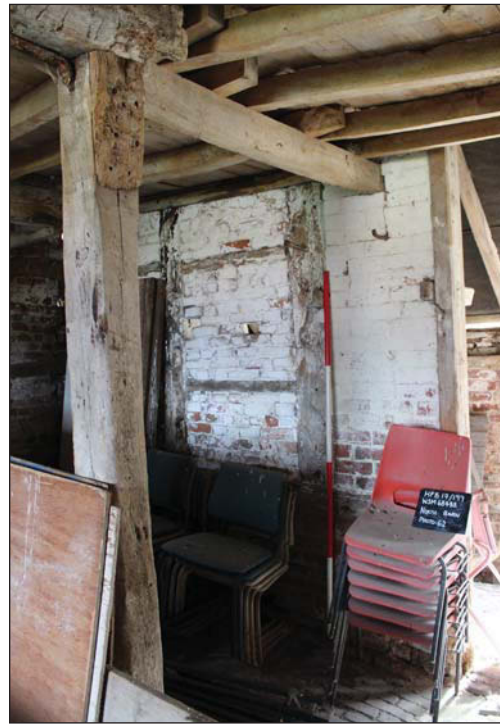
Plate 26. Interior, north barn, Bay 5, looking south east, Scales: 2m.
