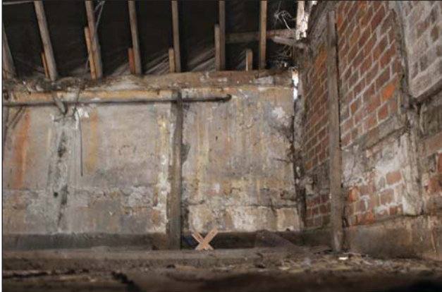
Plate 17. Interior, first floor (FF1) from Bay 1 stairs to south wall.
