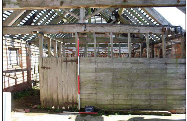
Plate 38. Exterior, north barn extension, Truss 1, looking east, Scales: 2m and 1m.
