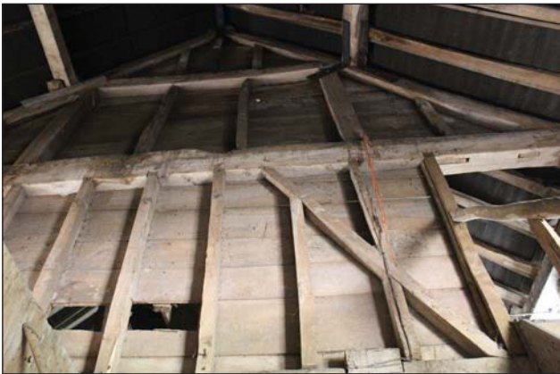
Plate 23. Interior, north barn, Bay 3, top of Truss 2, looking west.
