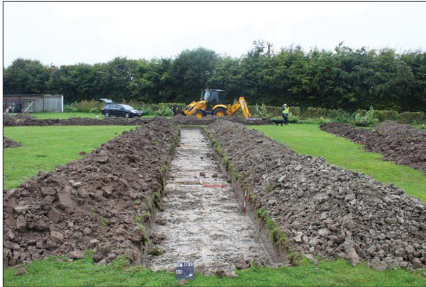
Plate 3. Trench 2, looking south-west, Scales: horizontal 2m and 1m, vertical 0.5m.
