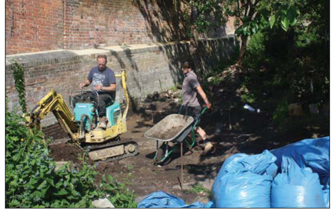
Plate 2. General view of office area, looking West.
