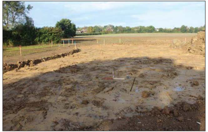
Plate 2. General view of stripped area, looking West. Scales: 2m and 1m.
