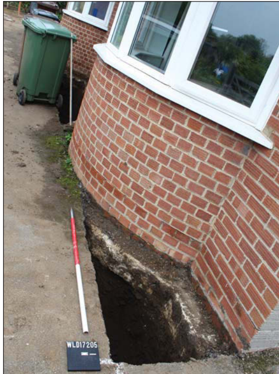
Plate 1. New footing, looking east, Scale: 1m.
