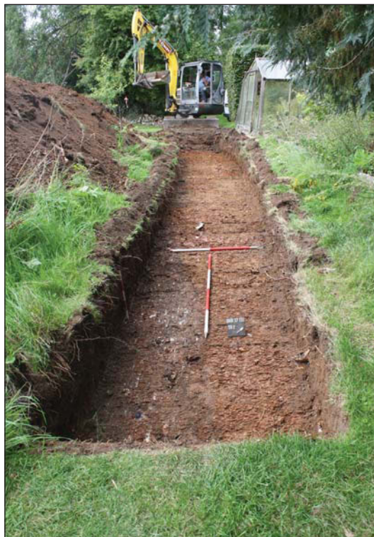
Plate 2. Trench 2, looking northwest, Scales: 1m and 2m.
