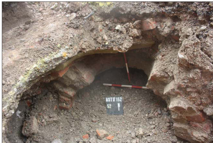
Plate 1. Culvert 52, looking north, Scales: 0.5m and 0.3m.
