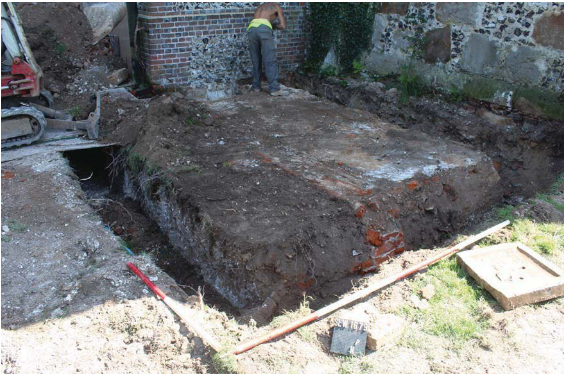
Plate 4. New footing, looking south east, Scales: 2m and 1m.
