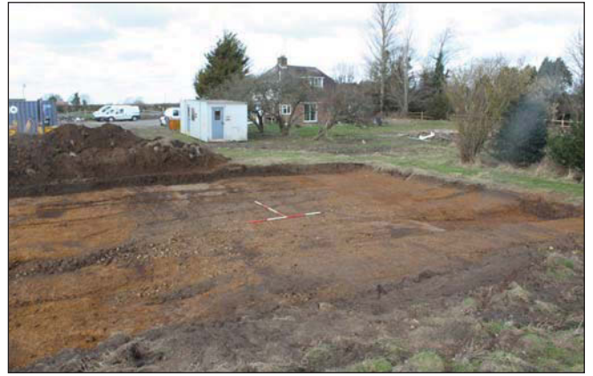
Plate 2. Road 57 after stripping, looking West. Scales: 2m x 2.
