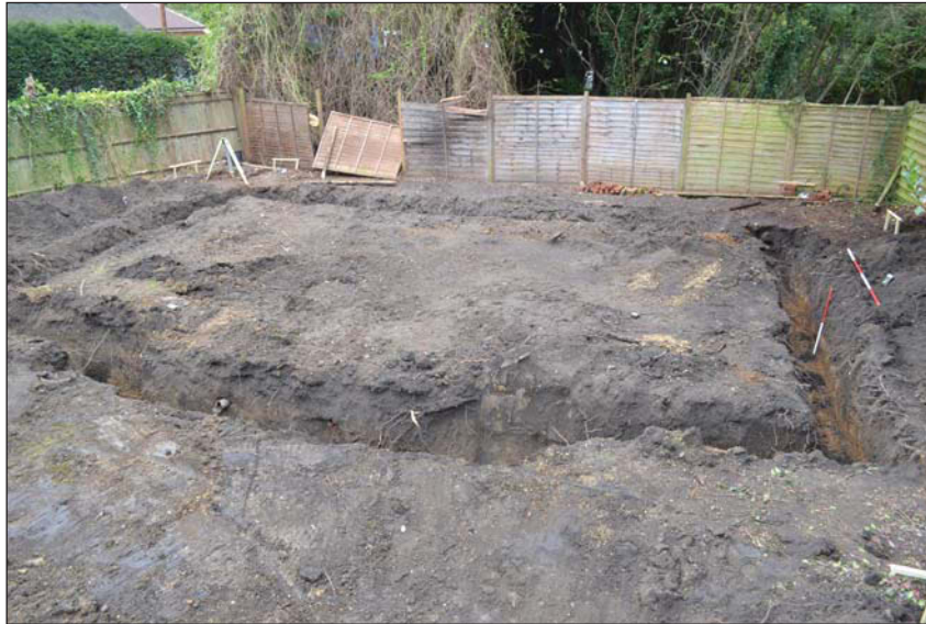
Plate 1. New footing, looking north east, Scales: 2m and 1m.
