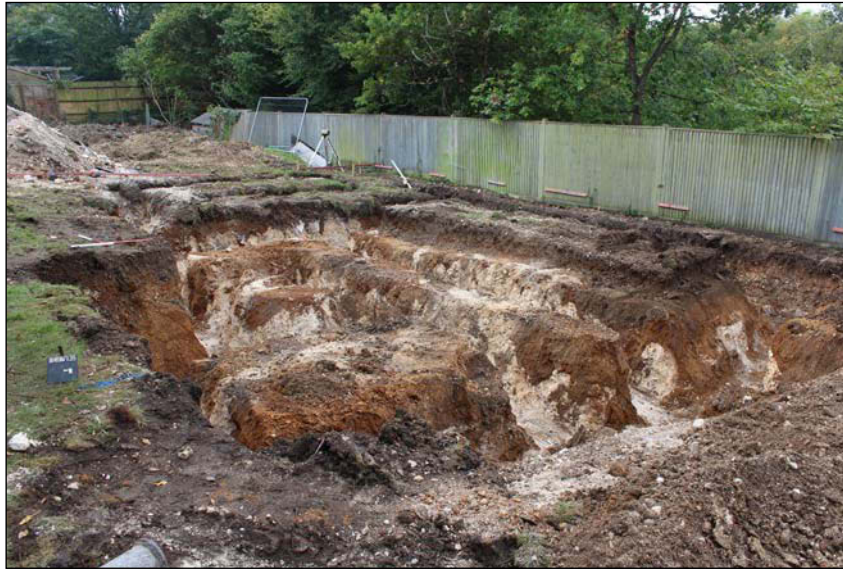
Plate 1. Overview of footings, looking north west, Scales: 2m and 1m.
