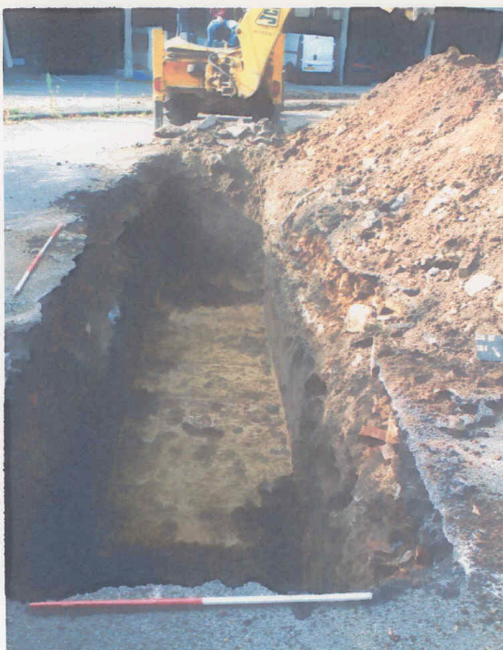
Plate 1. Trench 4 looking south west, far scale 2m; near scale 1m.
